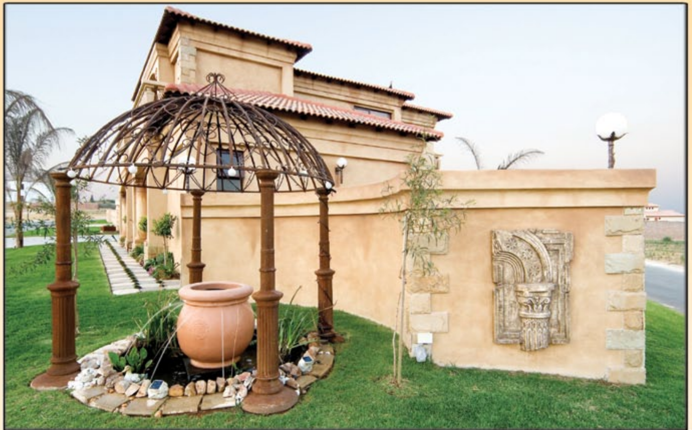
Roman Plaster combines well with natural stone cladding and wall features to achieve a Sicilian rustic appearance.
