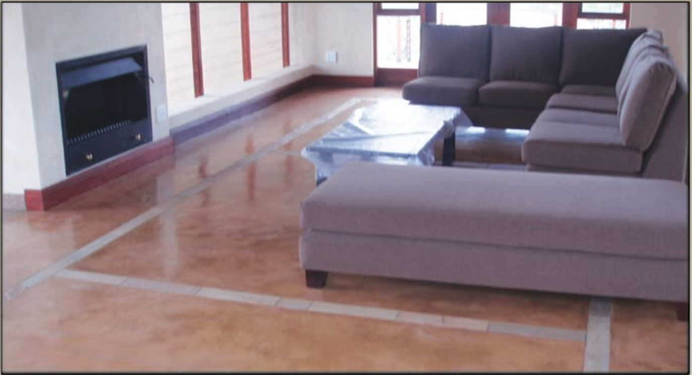
SL Floor Hardener is used on this floor in conjunction with natural, honed listello border tiles to lend a warm, rustic effect to this home's lounge area.
