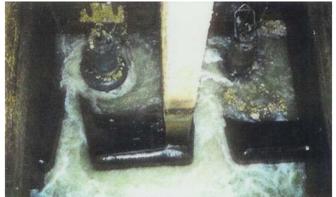
Self-cleaning action occurs at end of pump cycle
