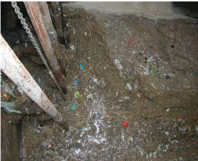
Accumulation of material floating on surface of sump
