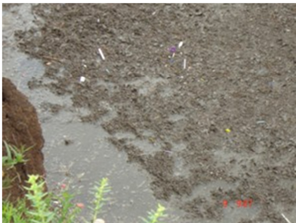
Notice that there is no sludge between the sludge bulk and the wall of the trench
